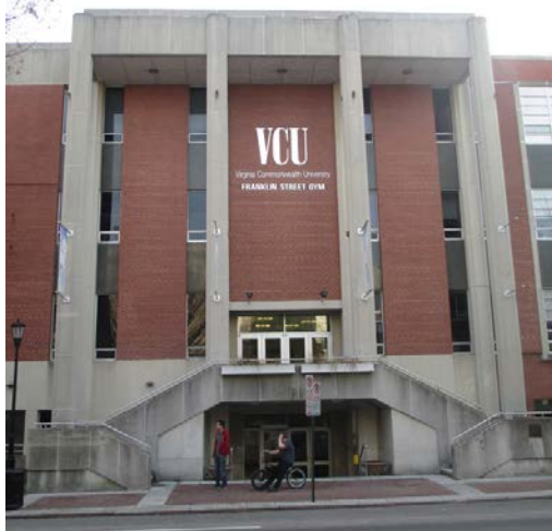
Franklin St. Gymnasium, Richmond, Virginia
